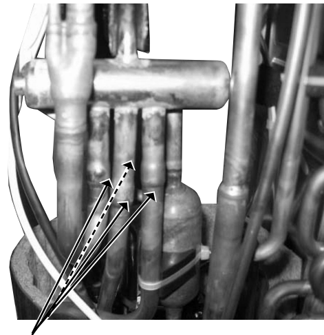
Welded parts of 4-way valve
